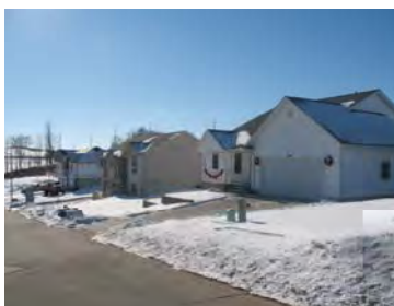
Region XII is completing three Speculative Homes in Conjunction with DMACC
